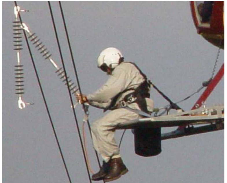
InterPhase Spacer installation from Helicopter using Barehand/Live Line work method
