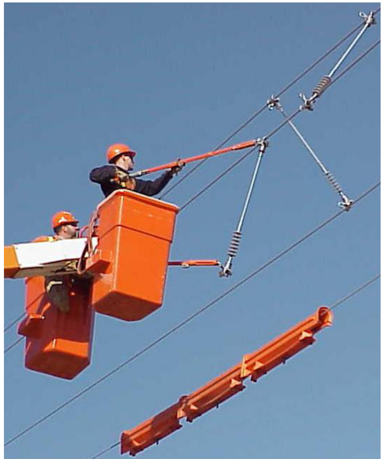
InterPhase Spacer installation using Hot Line Tools
