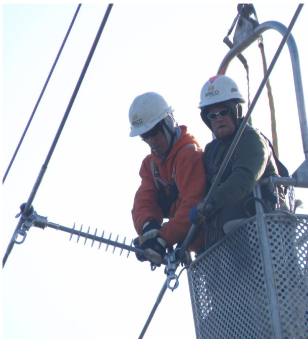
InterPhase Spacer installation
