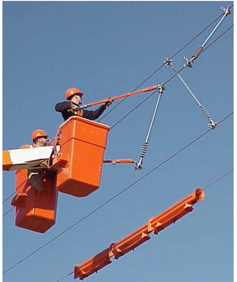
InterPhase Spacer installation using Hot Line Tools
