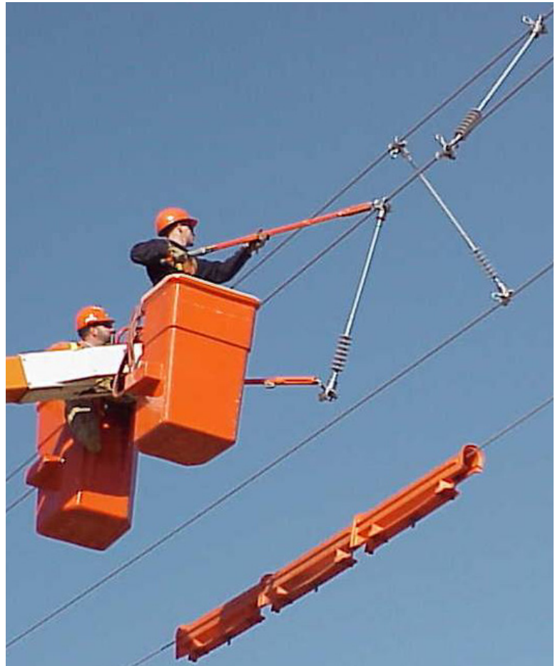
InterPhase Spacer installation using Hot Line Tools
